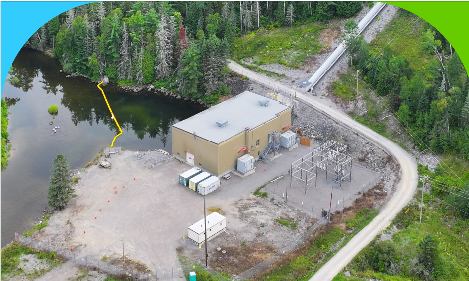
Original Matabitchuan GS site prior to demolition.
