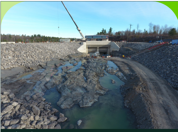
(Above) November 2022. Forebay, also known as the Headpond, is getting closer to watering up.
