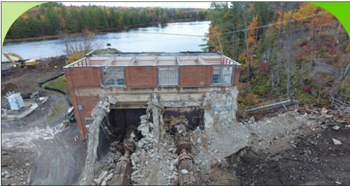
(Above) October 2020. During the demolition process of the former Calabogie Generating Station, its two turbines were extracted from the powerhouse.
