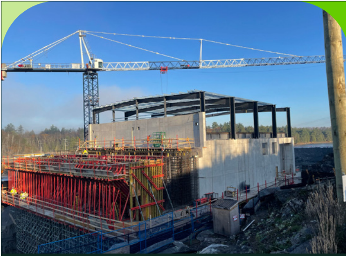
(Above) November 2021. Foreground - Intake passageway and deck concrete formwork being erected upstream of the powerhouse. Background - Powerhouse steel skeleton roof seen beneath crane boom.
