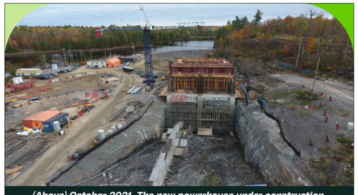
(Above) October 2021. The new powerhouse under construction, including a wider and deeper forebay to accommodate more flow through the units.
