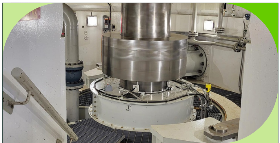
(Above) A look at the completed Unit 4 turbine pit at Barrett Chute GS.
