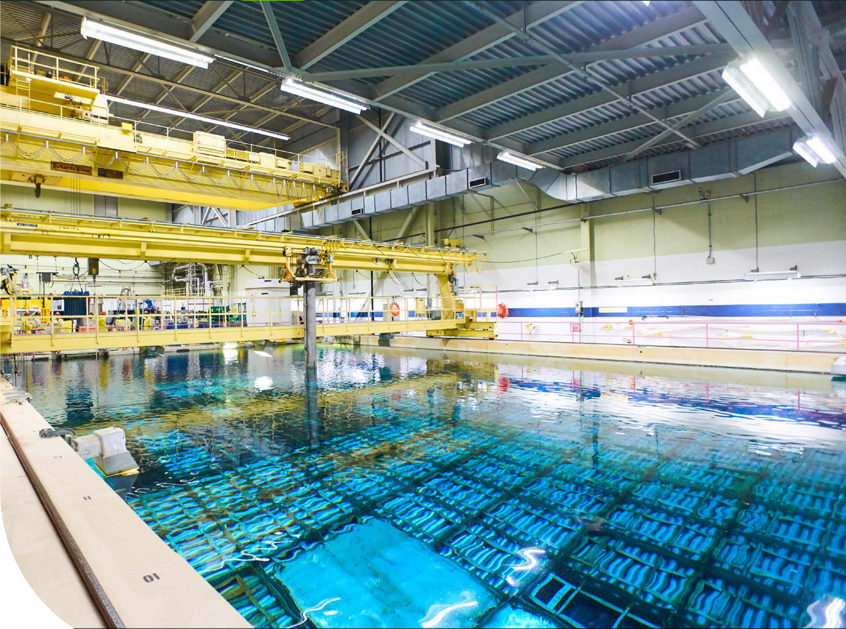
A look at the spent fuel pool at Pickering Nuclear Generating Station, where Cobalt-60 isotopes are stored and harvested.
