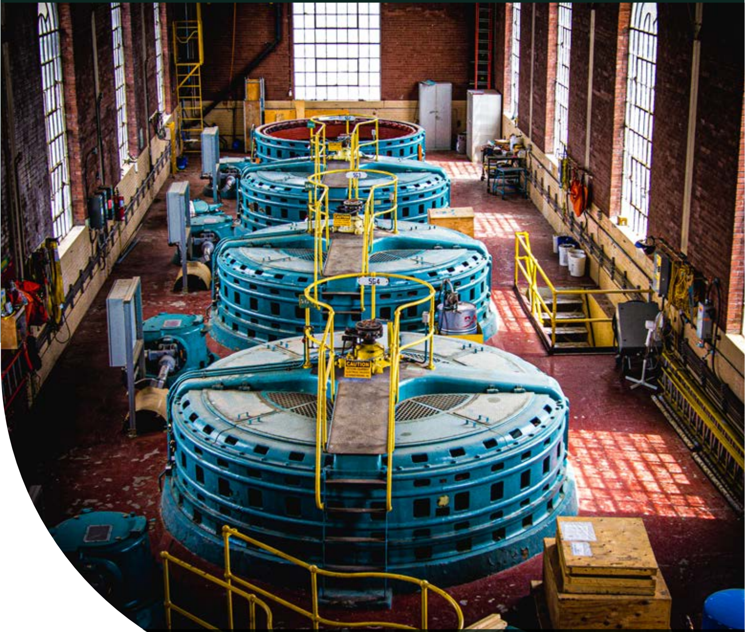
Generating units at an OPG hydroelectric station.
