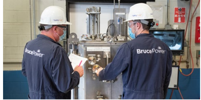
Bruce B's Unit 7 will be the first commercial reactor in the world able to produce Lu-177 and potentially other short lived medical isotopes. Operators train on a pneumatic system which delivers and retrieves the pencil-sized targets to the core of the reactor.
