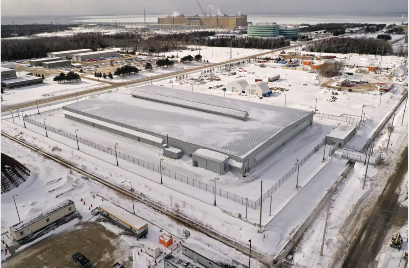
A new storage building was constructed in 2021 on the Bruce Site at OPG's Western facility to store used fuel from Bruce A and B.
