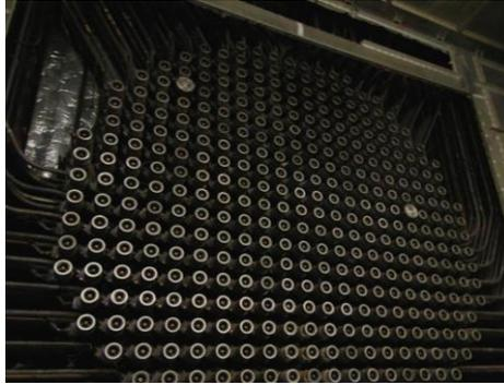
*Figure 2 - Reactor Face showing Fuel Channel End Fittings*
