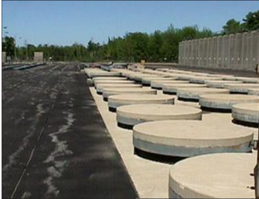
Figure 2-12: Cover Plates and Shield Plugs of IC-18 In-Ground Containers
