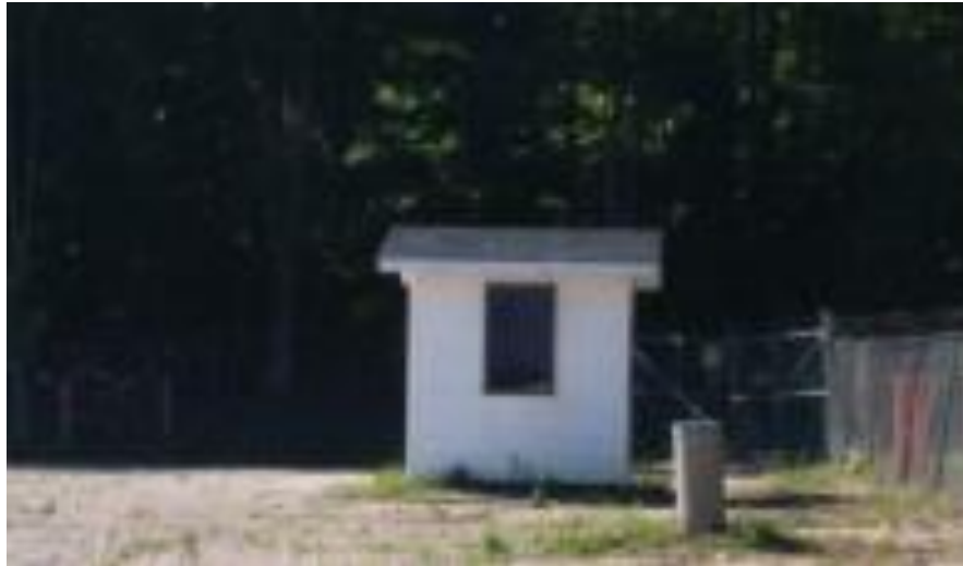
Figure 5-2 – RWOS1 Facility Temporary Shed
