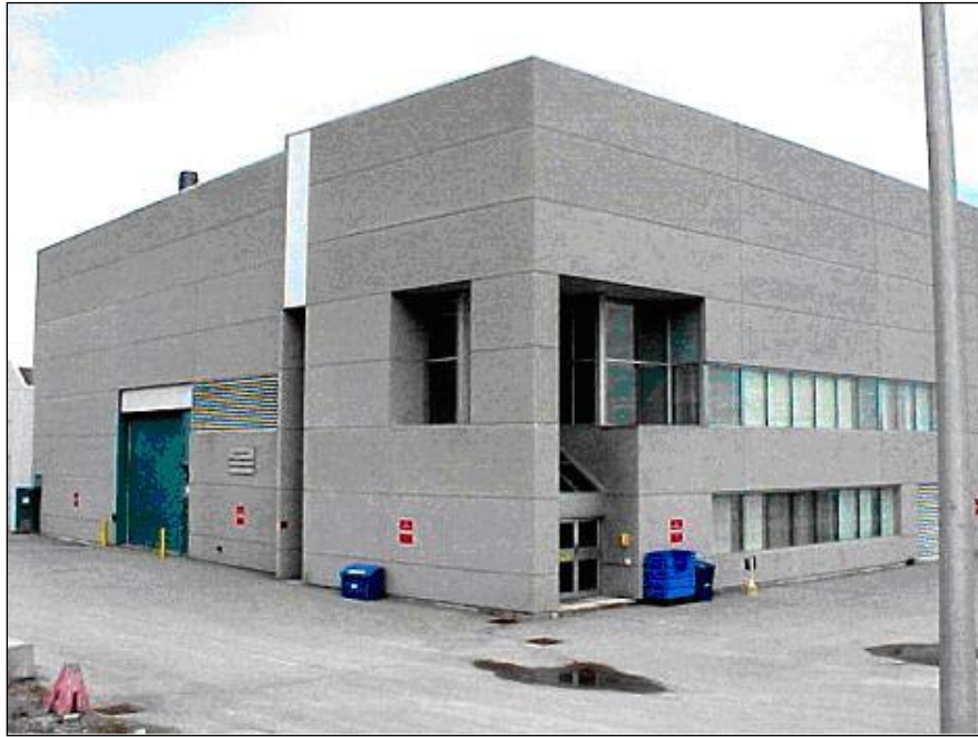
Figure 2-8: DSC Processing Building (Phase I) – Exterior
