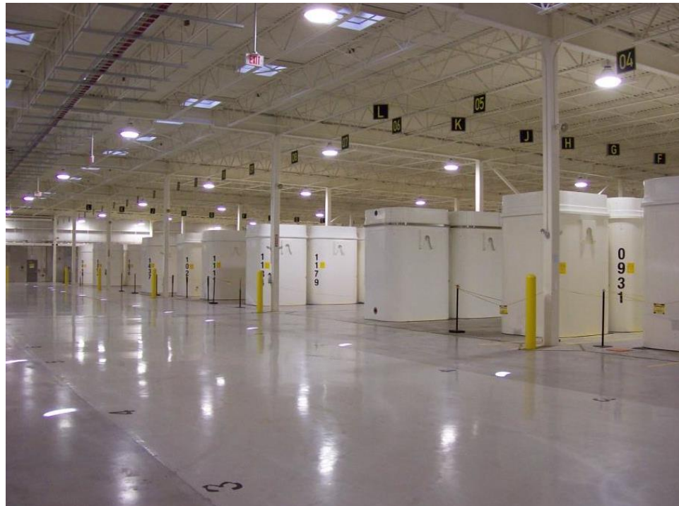
Figure 2-5: Dry Storage Containers in DSC Storage Building #1
