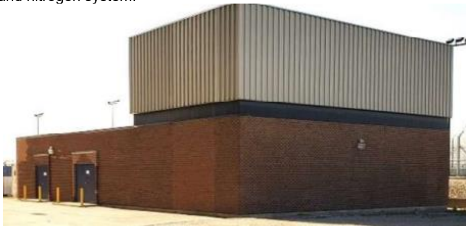
Figure 3 Off Gas Management Building
