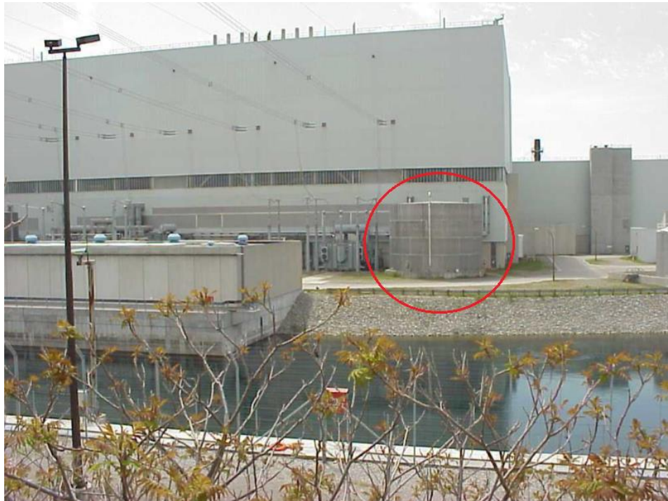
Figure 17 Demineralized Water Tank
