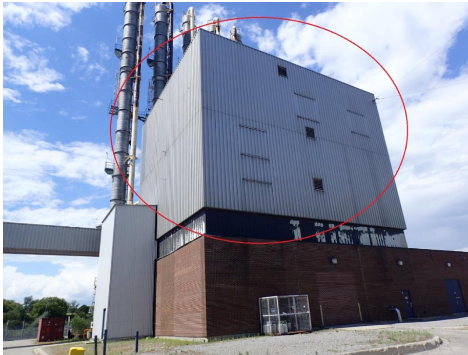
Figure 14 Heavy Water Upgrading Plant
