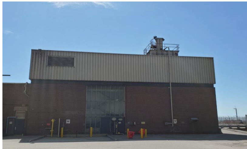
Figure 4 Old Water Treatment Plant
