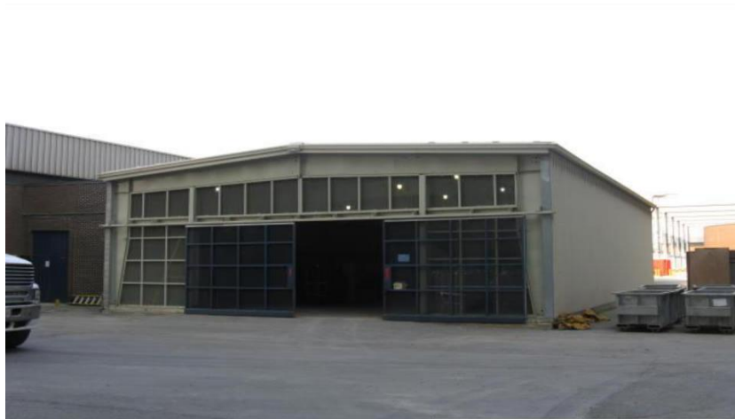
Figure 8 Gas Bottle Storage Enclosure
