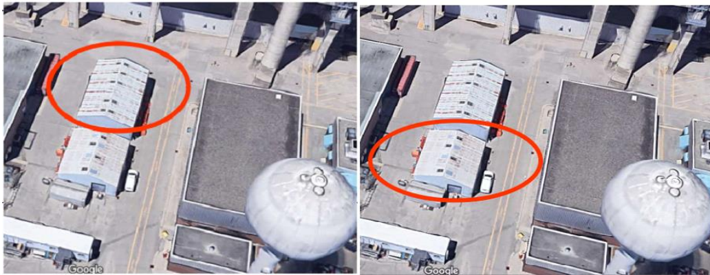
Figure 1 Scaffold Shed Buildings
