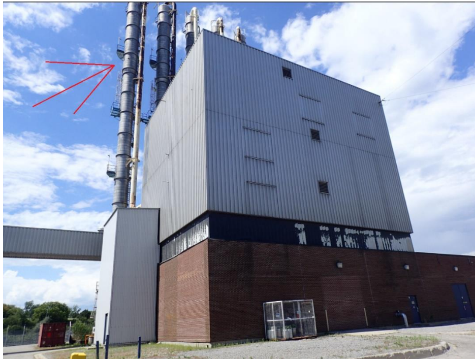
Figure 15 Heavy Water UPPA Upgrading Towers
