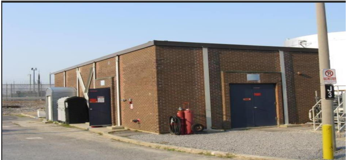
Figure 13 Standby Generator Pumphouse
