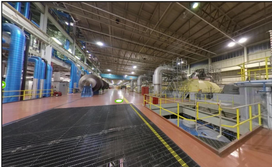
Figure 1 Turbine Hall 294' Elevation
