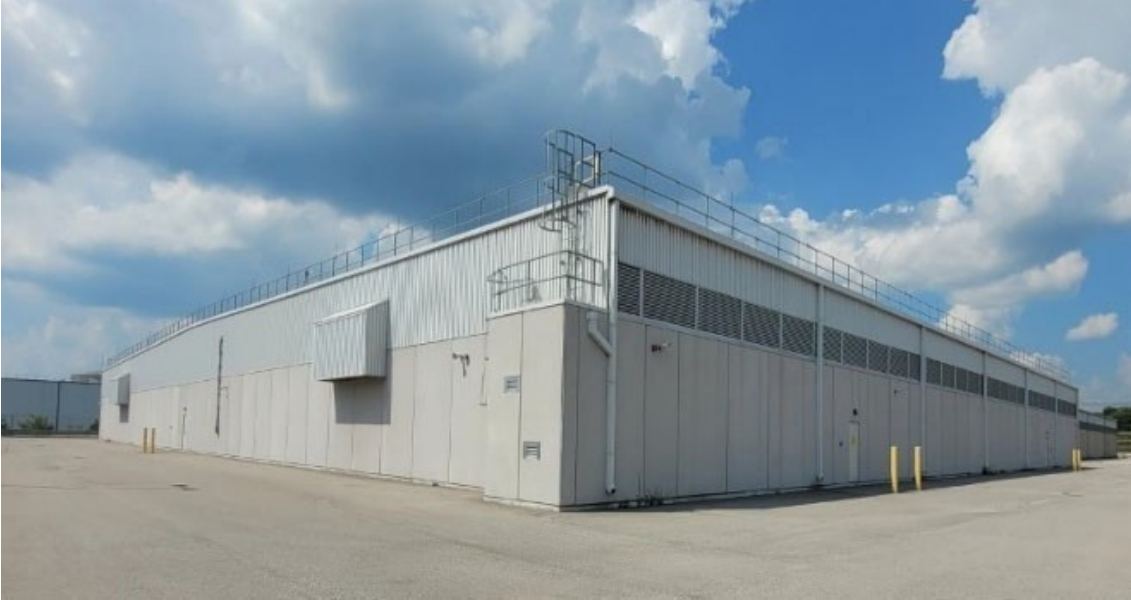
Figure 5: Used fuel Dry Storage Building #2
