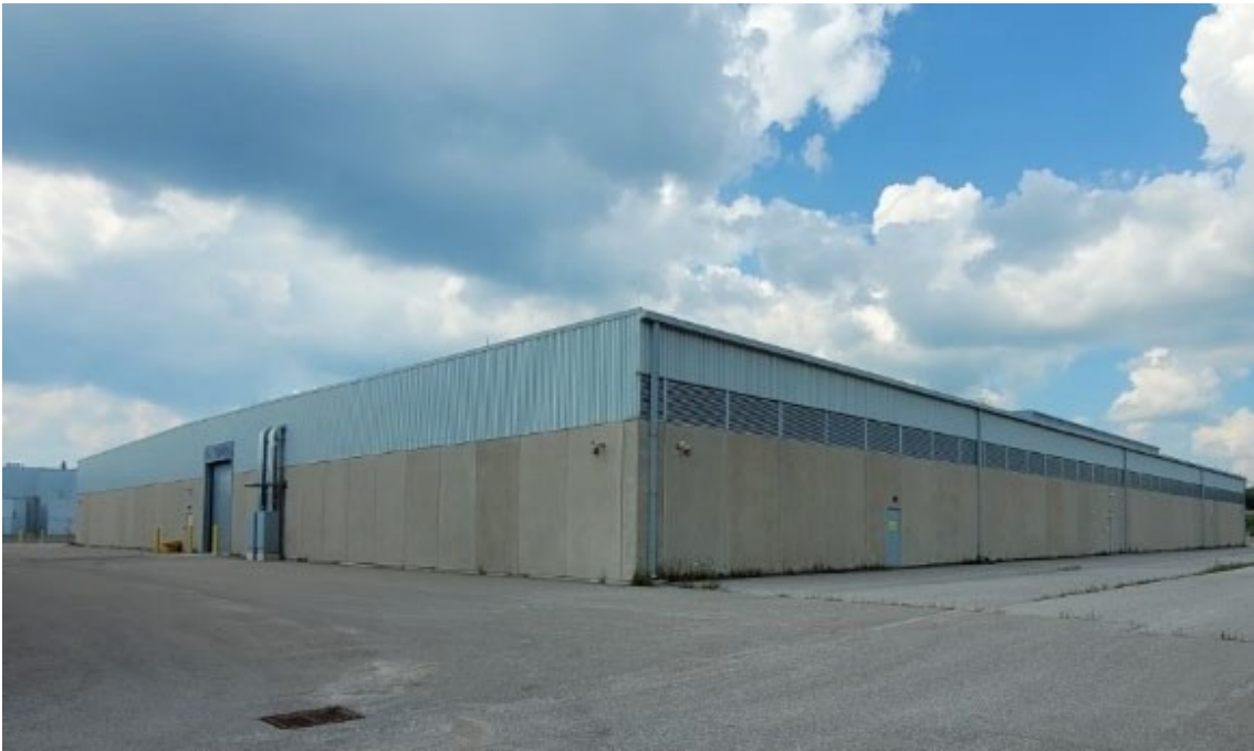
Figure 4: Used fuel Dry Storage Building #1
