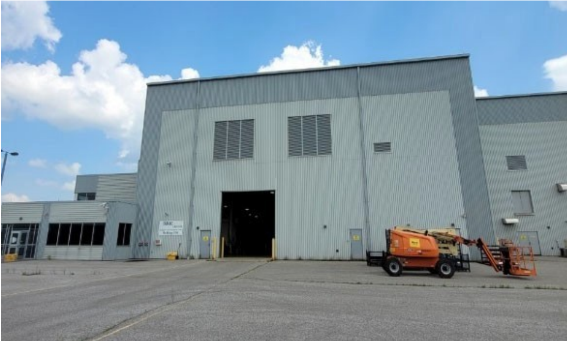
Figure 3: DSC Processing Building
