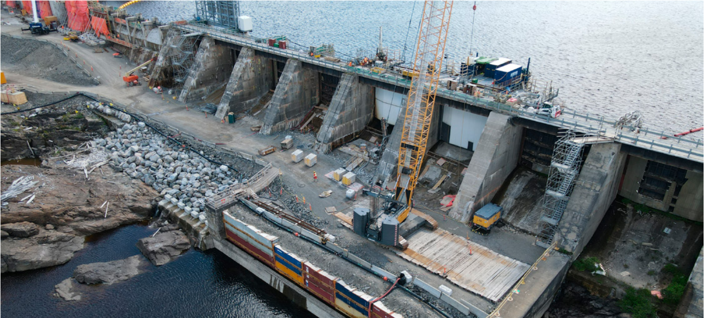
(Above) Smoky Falls gated spillway under construction with the downstream water retaining structure in place.
