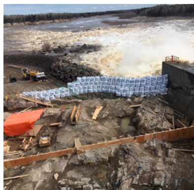
This drone photo highlights the excavation of the plunge pool on the downstream side of the sluiceway structure.
