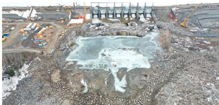
This drone photo highlights the excavation of the plunge pool on the downstream side of the sluiceway structure.
