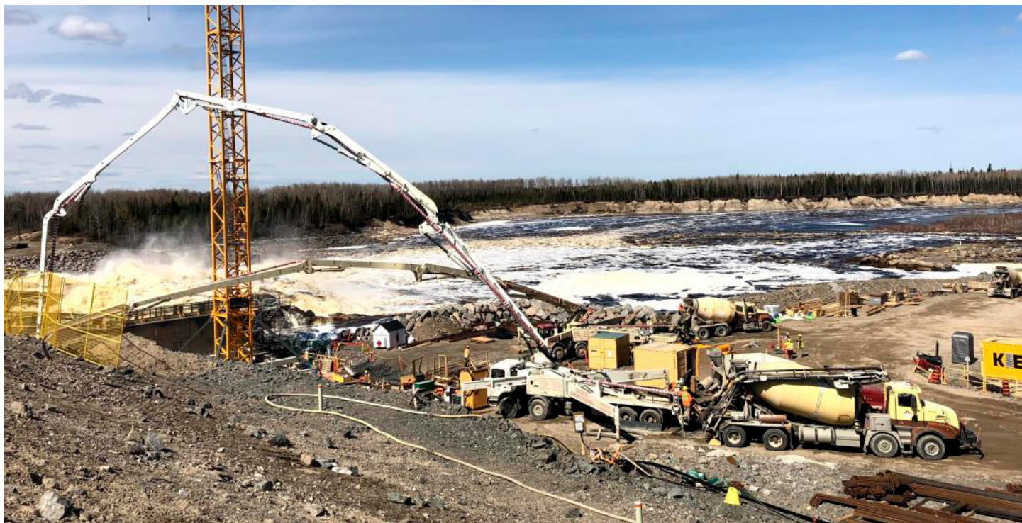
A tower crane is used to support construction on the east side of the Adam Creek sluiceway structure, part of the Little Long Dam Safety (LLDS) project.
