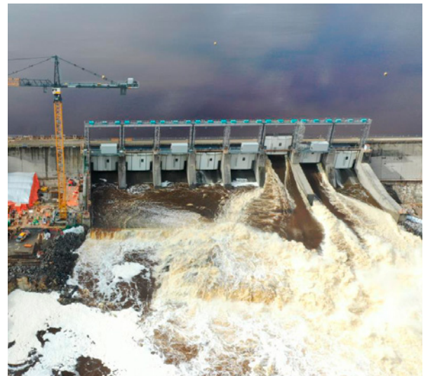
Although drier than normal conditions led to lower than normal freshet flows, Adam Creek sluiceway structure remained essential in diverting water to protect assets downstream.
