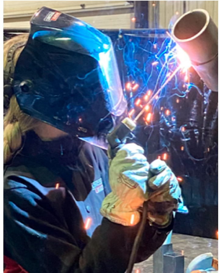
(Above) Megan Parent gains valuable experience working in industrial construction and repair.
