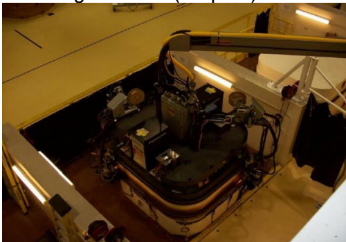
Welding Machine (Step 13)
