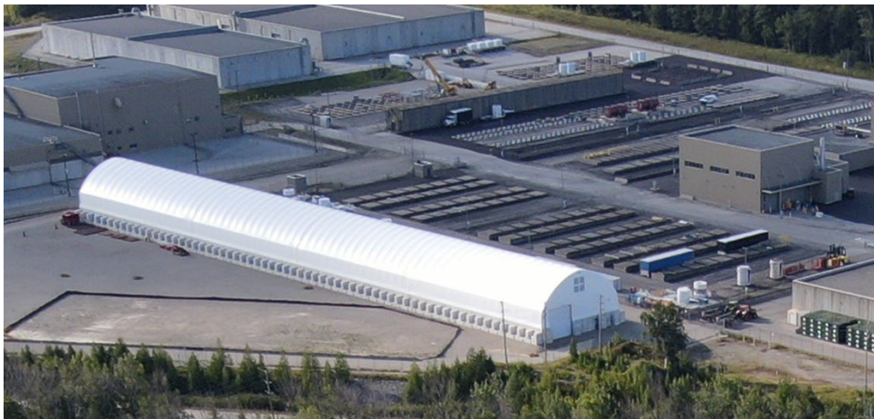
Figure 18: Multi-Purpose Storage Building
