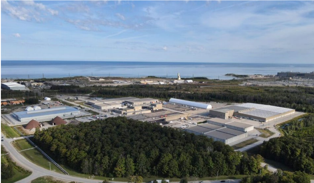
Figure 3: Western Waste Management Facility
