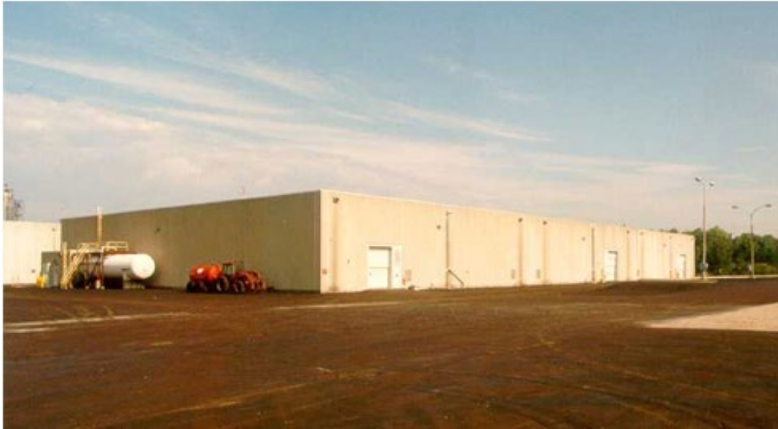
Figure 14: Low Level Storage Building
