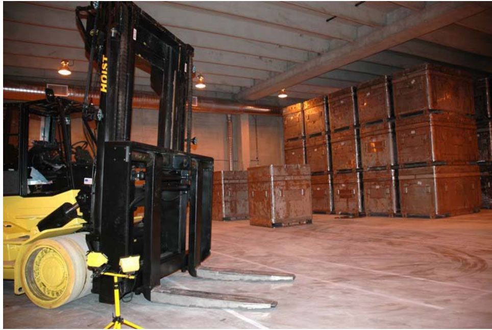
Figure 17: Retube Waste Container Storage at WWMF
