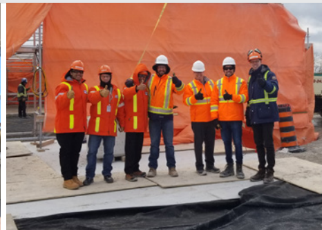
Pickering storage building foundation completed
