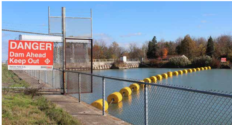
Warning signs, fences, booms and other barriers indicate hazardous areas to stay clear of. Pictured: DeCew Falls Generating Station
