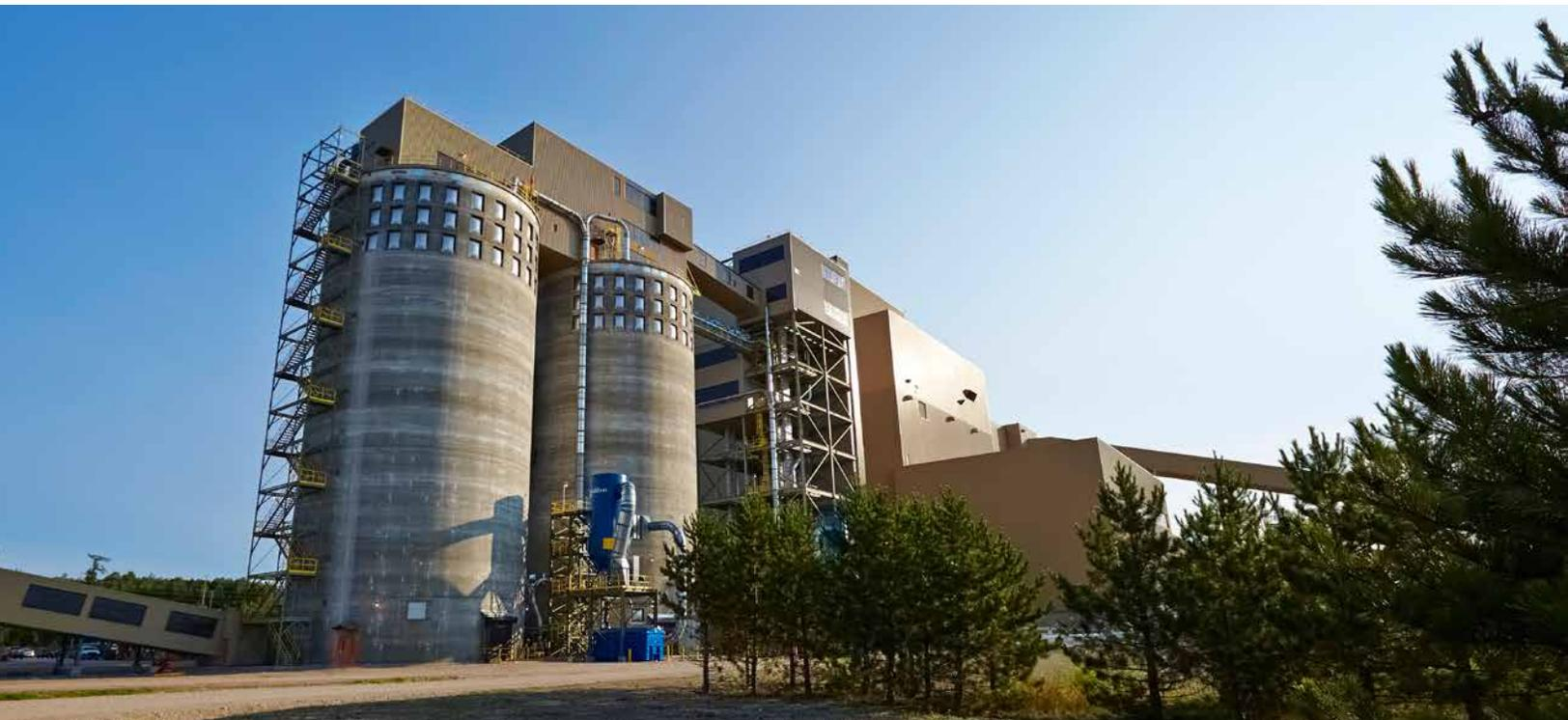
Two new silos were constructed at Atikokan during the conversion to biomass. Each is 44 meters tall, and holds approximately 5,000 tonnes of wood pellets.
