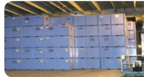
Low level waste containers inside a licensed facility.
