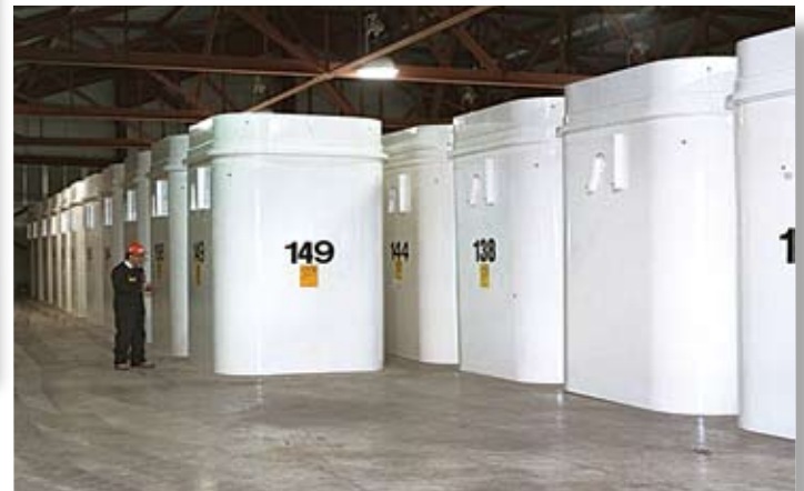
Used nuclear fuel dry storage at the Pickering Waste Management Facility
