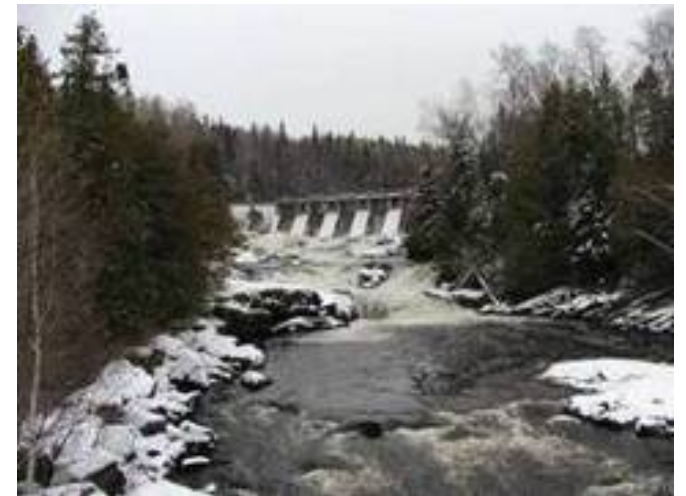
Mattagami Lake Control Dam
