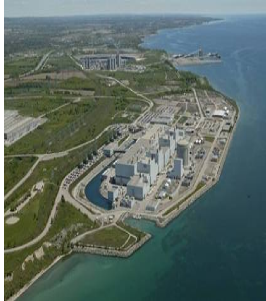
Darlington Nuclear Generating Station
