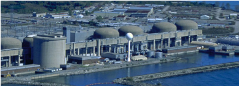
Pickering B Nuclear Generating Station
