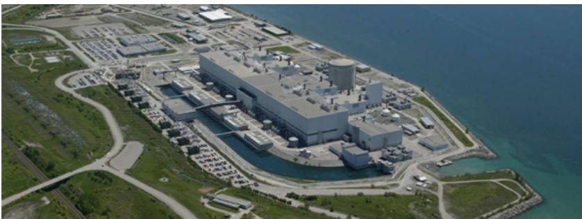
Darlington Nuclear Generating Station
