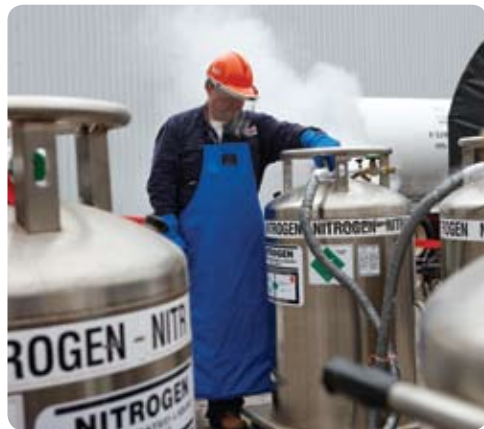
A member of the VBO’s “ice plug” crew freezes a portion of pipe. Pipe freezing enables maintenance and repair work on systems without the need to cut piping.
