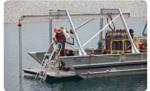
A diver prepares to enter the water to inspect a part of the ESW system. During the outage, zebra mussels were found to be impeding water flow in the cooling water supply lines. Divers helped remove over 520 tonnes of zebra mussels, restoring flow well above requirements.
