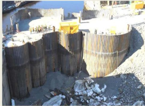
Lower Mattagami Hydroelectric Project
